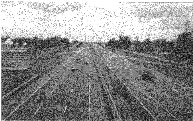
The Lake County Engineer took a lead role in conducting the Major Investment Study for SR-2 (above), which was completed in a record 15 months.
